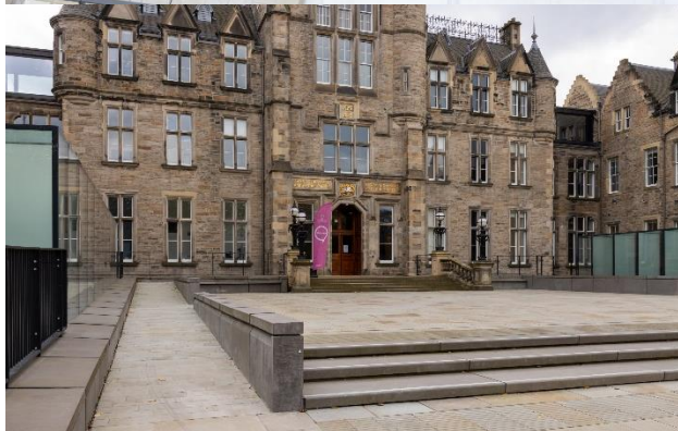
Ramp at Edinburgh Futures Institute. Original stone staircase moved forward to accommodate ramp. Category A listed, LB30306, 31/05/1994.
