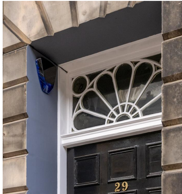
Good example of a sensitively positioned security alarm box on ingo of doorway.
