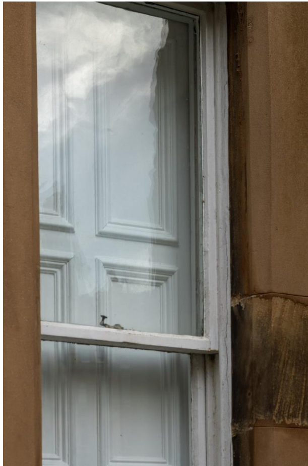
Example of timber window shutters seen from the outside.
