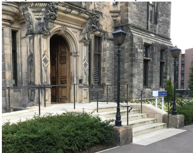
Good example of handrail design at St Leonard's Hall, Category A listed, LB28619, 12/12/1974.
