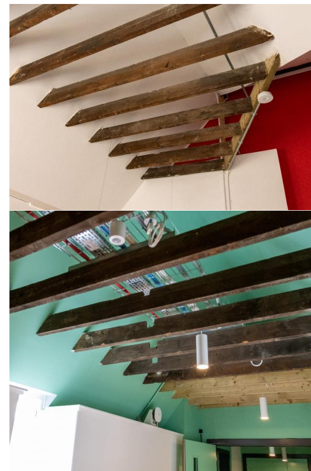
Surface mounted services behind original roof beams.
