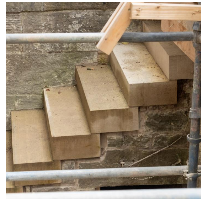
Repair being made to basement stairs.
