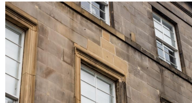
Indent stone repair and matching window details.
