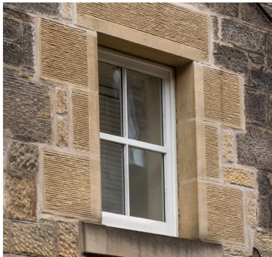
Matching stonework around new window.
