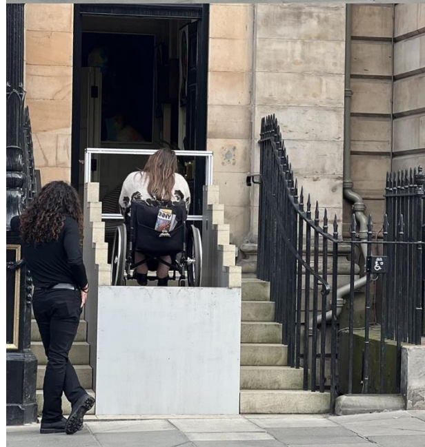
Hidden platform lift in use. Stairs fold back to form the platform and the lift provides level access for the user.
