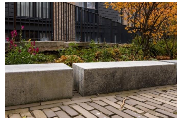
Public realm seating with channel to allow drainage into adjacent rain garden.
