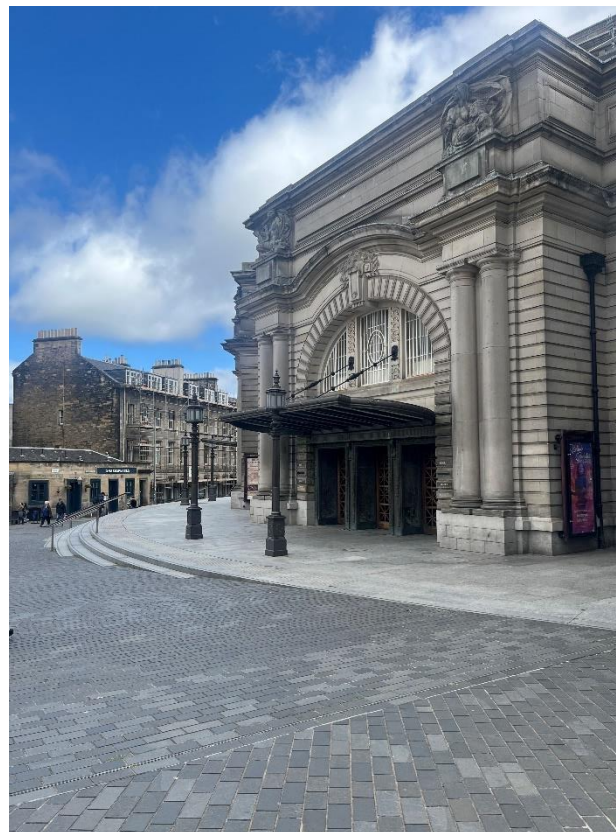
Regrading of ground at the Usher Hall to provide a level entrance, Category A listed, LB27780, 14/12/1970.
