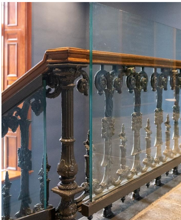
Safety barriers retrofitted to original features.
